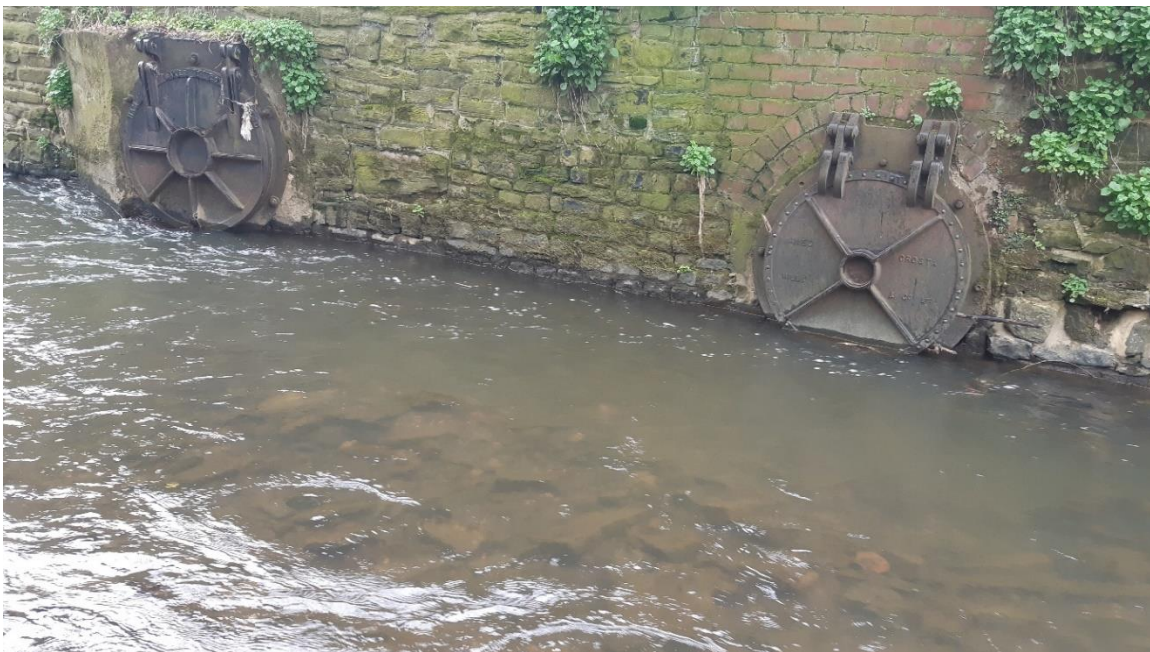
Figure 18: Paired outfalls at 53.355833, -1.483889. Discharges can be within consented values while still having a negative ecological impact. However, when it comes to discharges outside of consented values, the vigilance of members of the Sheaf and Porter Rivers Trust could be highly significant. At a basic level, ensuring discharges are consistent with extreme rainfall rather than unregulated discharges during dry weather helps to identify potential problems.
