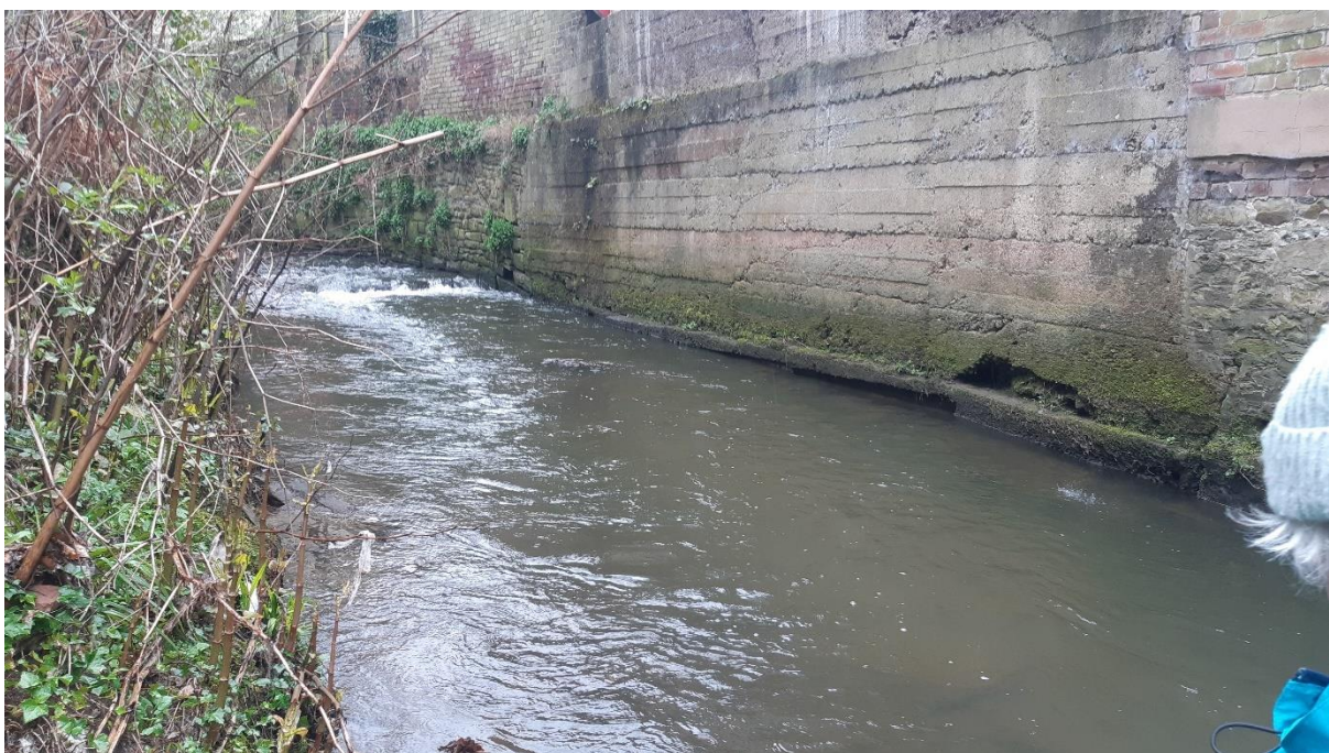
Figure 16: Japanese knotweed on the RB and gradual erosion of stonework on the LB.
