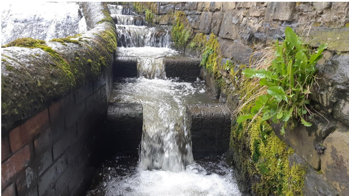
Figure 30: While much more passable than the weir, finding and negotiating this fish pass will be a significant challenge for all species of fish.
