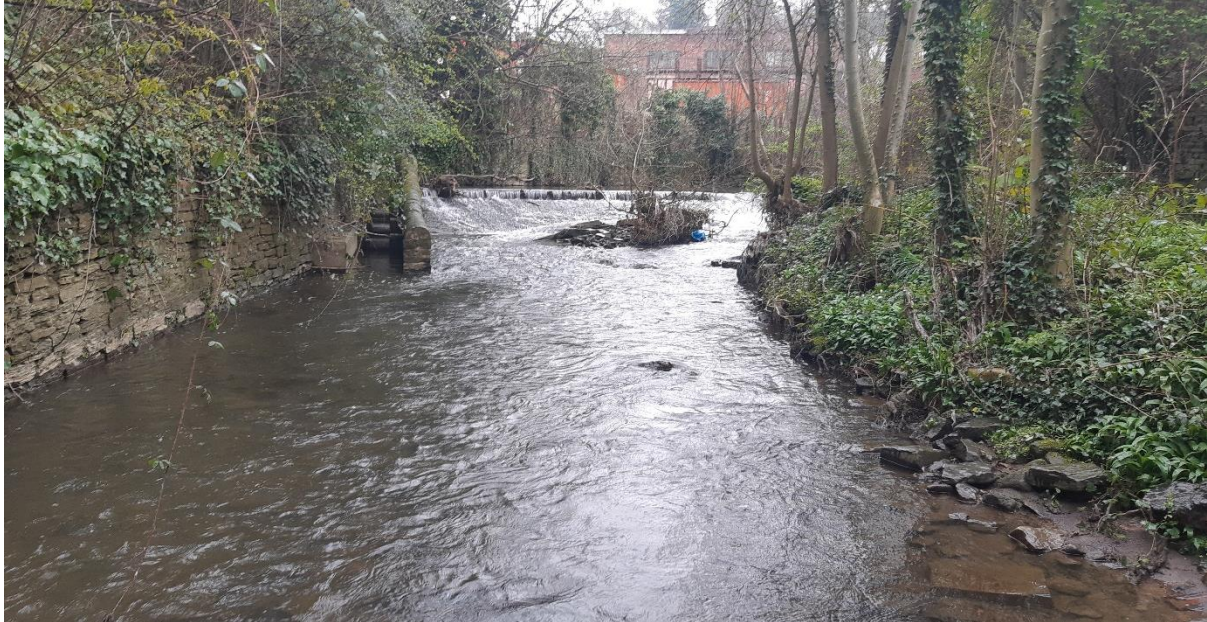
Figure 19: Stone weir with blocked fish pass on the RB and vegetated cobble bar feature on the LB.
