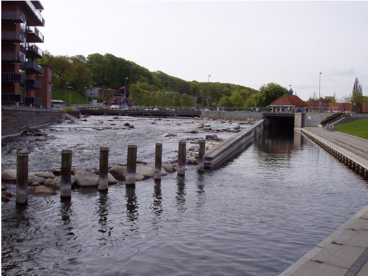
Figure 31: Rock ramp overcoming a large weir. Note that the use of stone substrate has created a nature-like riverbed which has inherent habitat value.
