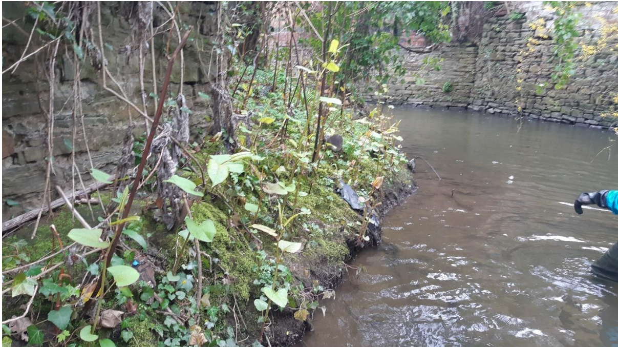
Figure 15: A more significant stand of Japanese knotweed putting the footings of this wall at risk as well as shading-out native riparian plant species.
