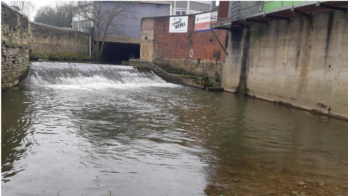
Figure 29: Weir defining the upstream limit of this survey at 53.351603, -1.484237
