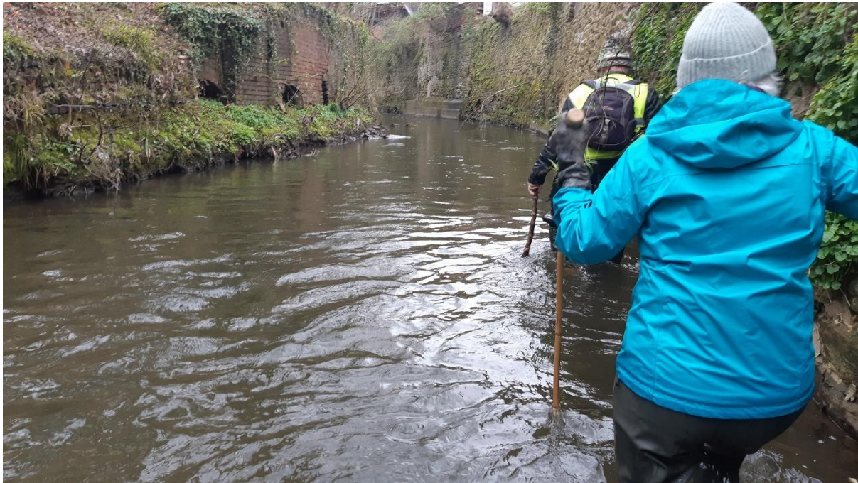
Figure 11: Walled, incised channel cut off from its floodplain with limited opportunity for riparian woodland growth. Locking the channel in place with stonework also prevents the natural migration of a river across its floodplain over time. This lack of temporal variation is highly significant and generally under-appreciated when compared to structural complexity. Washout of gravels is also likely within the confined, vertical-walled "chute".
