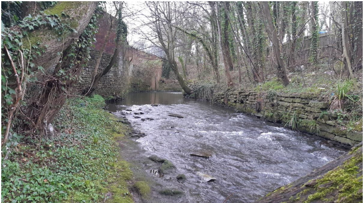
Figure 14: Pool, riffle and boulder-rapids sequence providing habitat variety in the face of multiple constraints. Every instance where even a short section of channel has its retaining walls set back from the channel results in the formation of a more natural, vegetated riverbank (left of frame, foreground).
