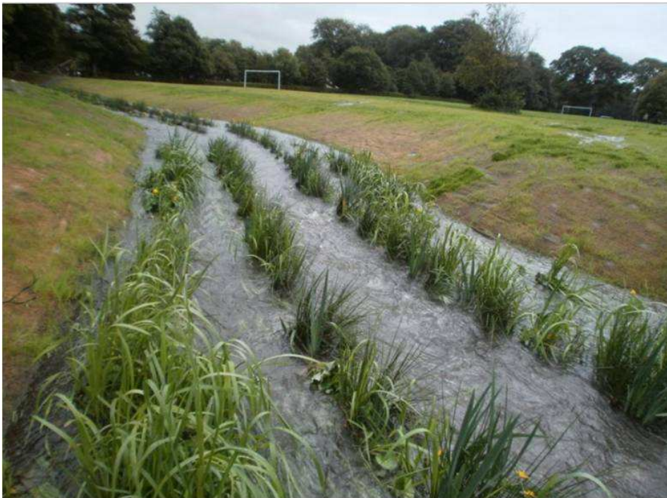
Photo 4: Post - The start of a flood event that eventually reached bankfull. Note the maturity of the vegetation installed just 6 weeks before. Immature coir rolls and pallets would have failed here.
