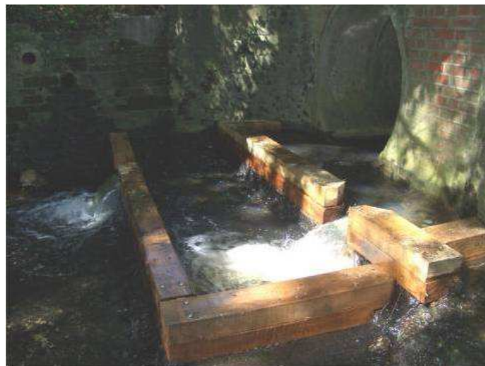
Figure 7: Simple "pre barrage" easement constructed by bolting wooden sleepers to the stream bed. For maximum efficacy - gently curved surfaces at the base of each slot are used to produce a solid "plume" of water for fish to swim up (cost £700).
