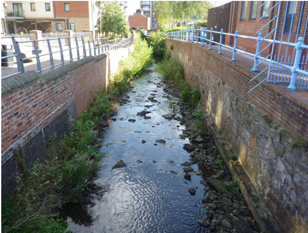
Figure 3: Reformation of a slightly meandering path via deposition of stream bed material transported from upstream reaches during spate flows. The valuable presence of marginal vegetation also owes its existence to this process. It is unusual to find this type of briskly flowing watercourse immediately upstream of a weir – and is a product of the steep gradient and relatively narrow confines of the channel.
