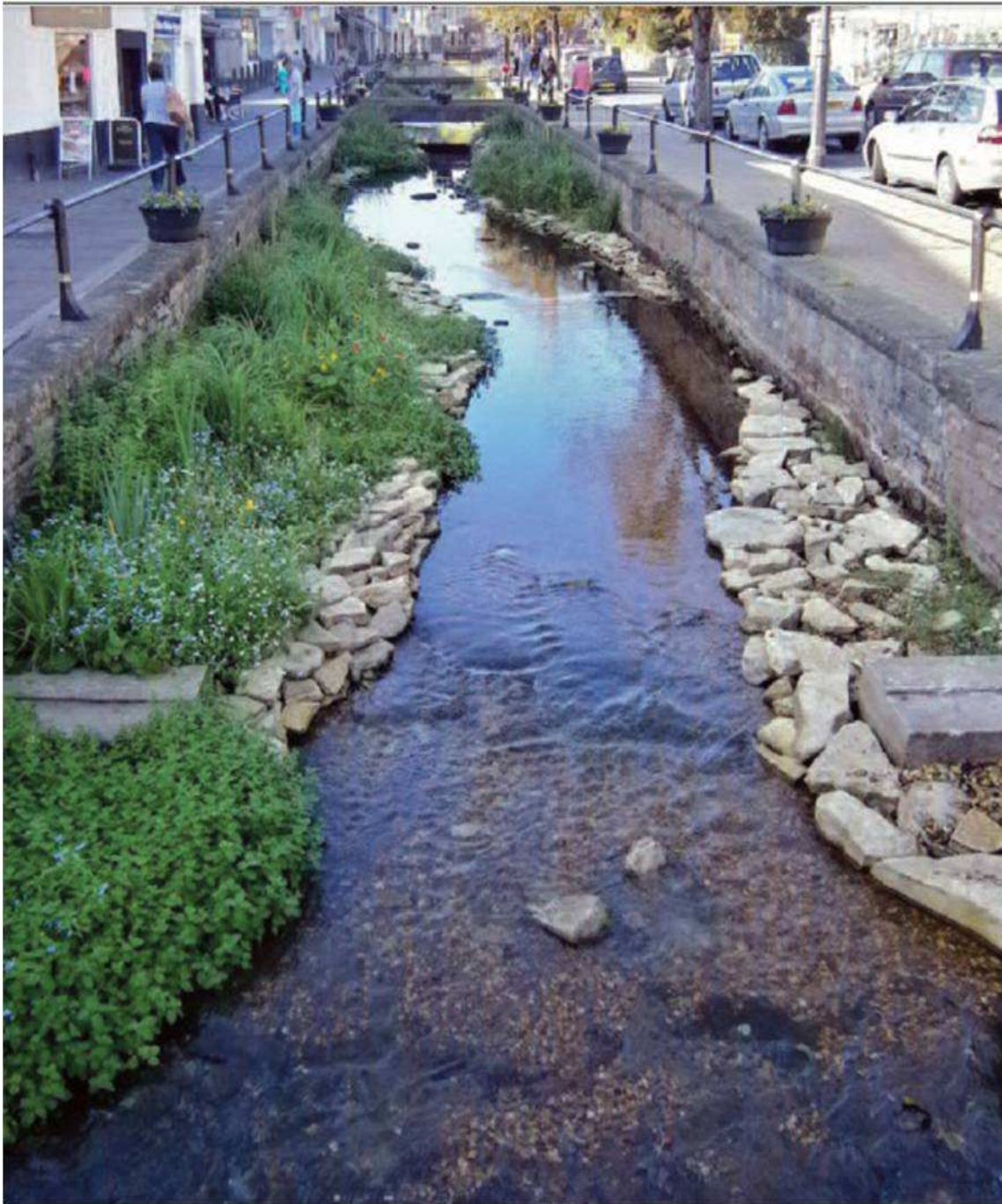
Figure 9: Meandering planform, aquatic plant establishment and introduced gravels/cobble substrate within retaining walls of an engineered channel.
