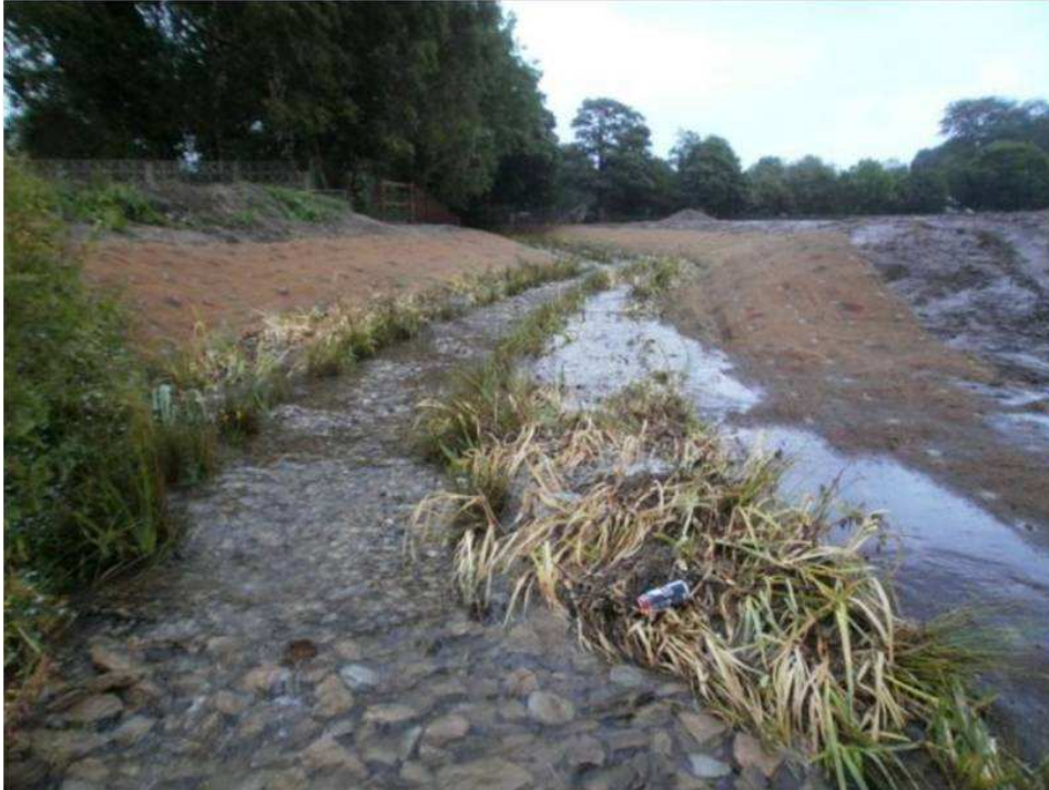
Photo 3: Installation - Mid July 2011
