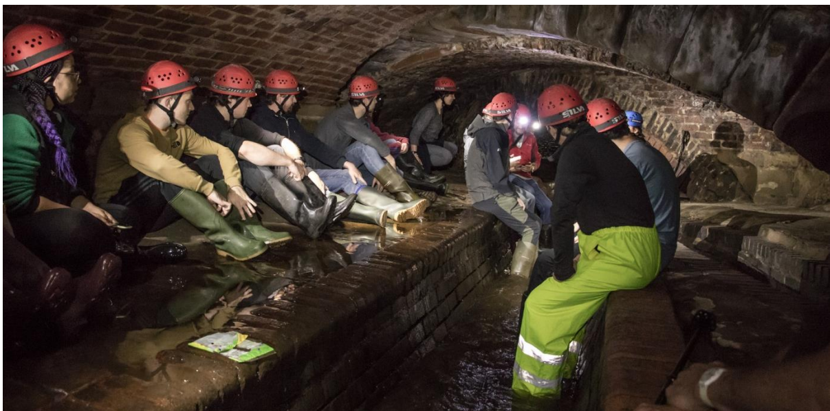
Figure 3: Brick-lined central “low-flow” channel of the Porter Brook where the Leadmill Stream joins along the RB.
