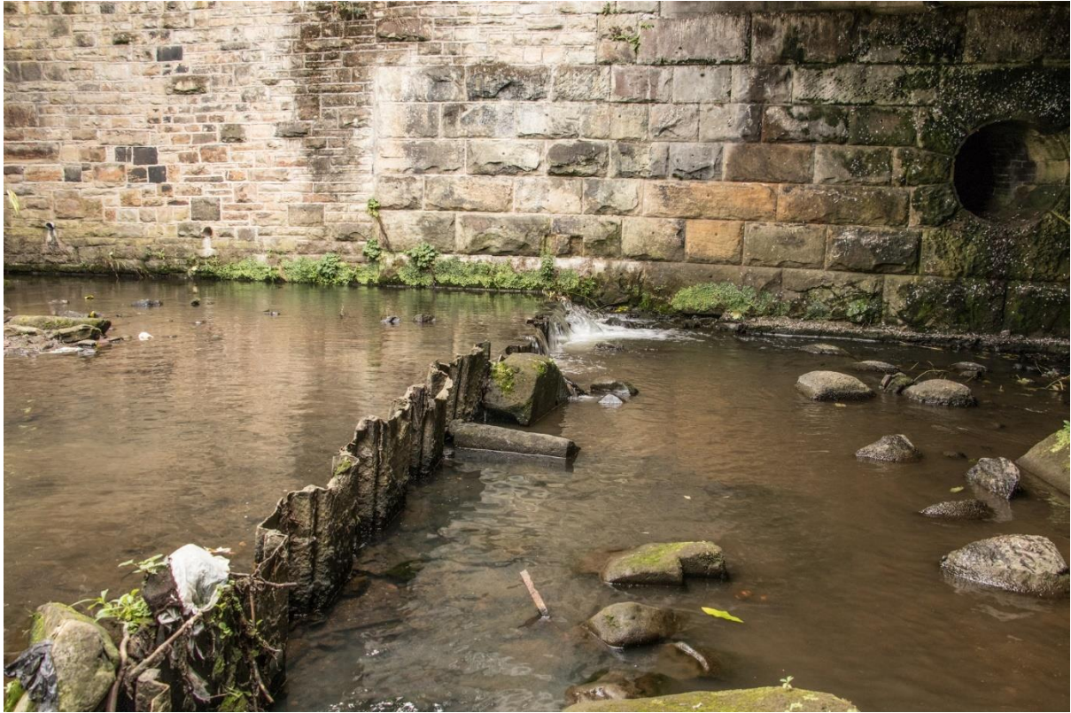
Figure 11: Sheet piling impounding structure and barrier to free fish passage.
