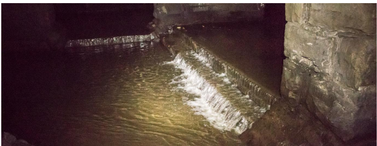
Figure 7: Although seemingly small and insignificant, the shallow water below this step prevents fish from being able to leap this barrier.
