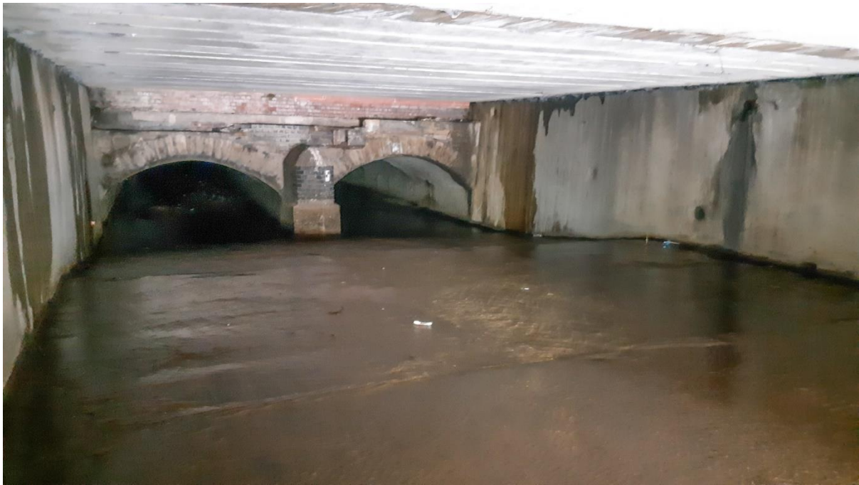
Figure 5: Laminar, uniformly-shallow flow down a sloping apron creates a significant obstacle to fish.
