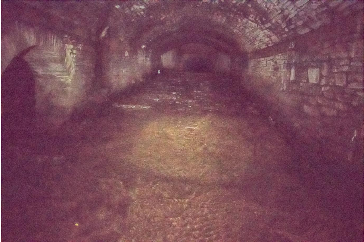
Figure 6: Although suffering from poor lighting, it is possible to note another sloping, shallow-water obstacle to fish movement at the confluence of the Sheaf and Porter
